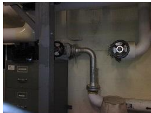
Figure 42 Conventional image of bare piping to hot water tanks.
