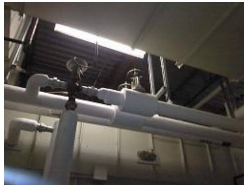
Figure 56 Conventional image of the same three way valve and bare bonnets.
