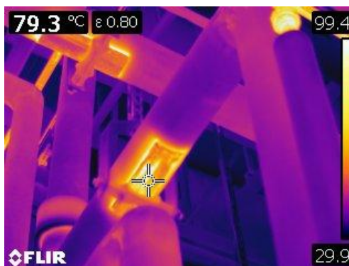
Figure11 This is a thermographic image of pipe supports without insulation behind them at 79° C or 174° F. (12 of)
