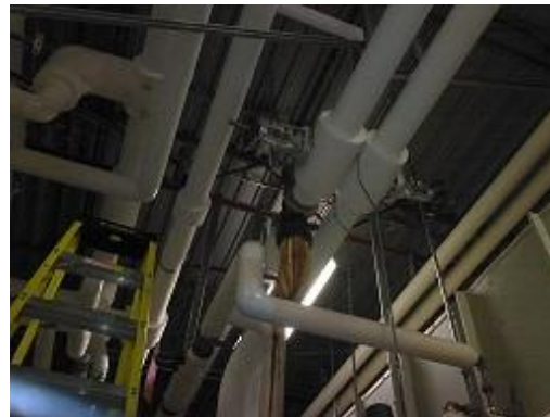
Figure 48 Conventional image of bare small bore heating supply and return to coils.
