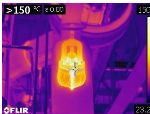
Figure 23 Thermographic image of a large bore bare valve bonnet at 140° C or 302° F.
