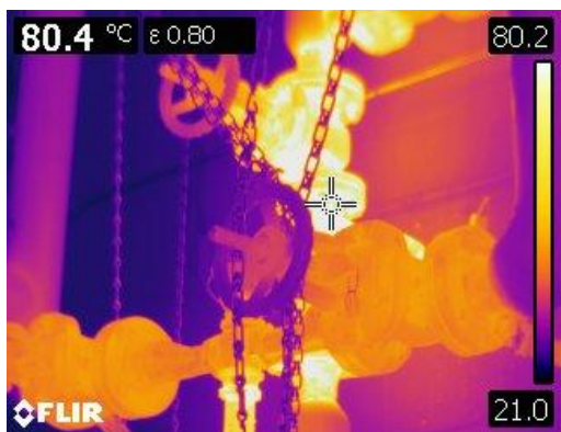
Figure 33 Thermographic image of heating supply pumps at 96° C or 204° F.
