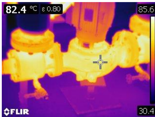
Figure 71 Thermographic image of bare motorized heating pumps at 82° C or 179° F
