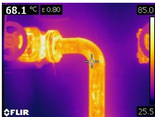
Figure 41 Thermographic image of bare piping to hot water tanks at 68° C or 154° F.
