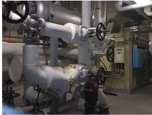
Figure 70 Conventional image of the same valve bonnets and damaged insulation .
