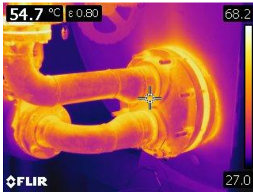
Figure 43 Thermographic image of bare piping and heat exchanger at hot water tanks at 54° C or 129° F.
