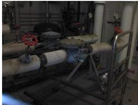
Figure 4 This is a conventional photo of the same pump. There are also an exposed valve spindles and unions.
