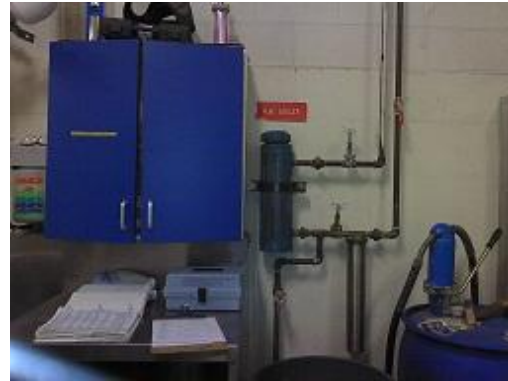
Figure 38 Conventional image of the chem. pot and associated piping.
