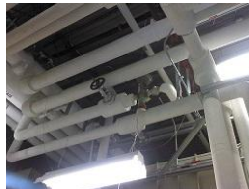
Figure 50 Conventional image of the bare three way valve and valve bonnet.
