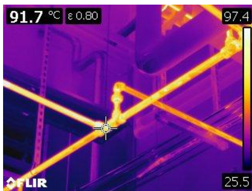
Figure 9 This is a thermographic image of bare 1 1/4 steam line in the boiler room at 91° C or 195° F. (over 40 ft)
