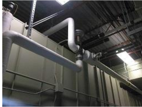
Figure 54 Conventional image of the same three way valve and bare bonnet.
