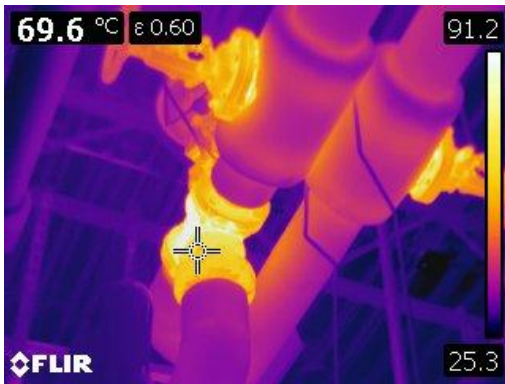
Figure 47 Thermographic image of bare heating supply to 69° C or 156° F.
