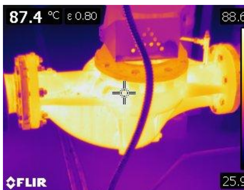
Figure 63 Thermographic image of bare motorized heating pump at 87° C or 188° F
