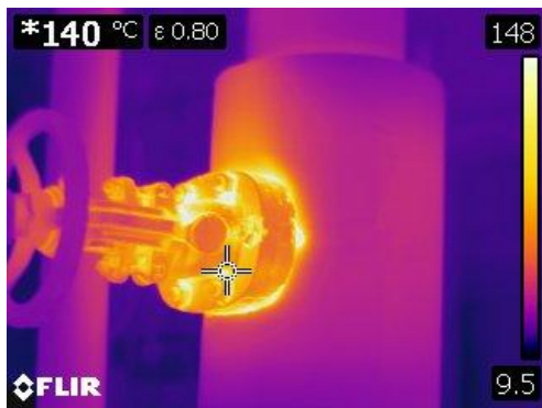
Figure 7 This is a thermographic image of a bare valve bonnet at 140° C or 284° F.
