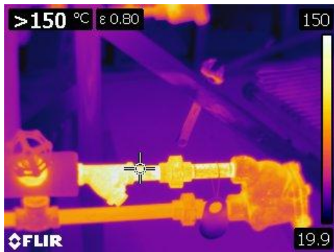
Figure 5 This Thermographic image of a steam trap and piping below the previous valve assembly at 150° C or 302° F.
