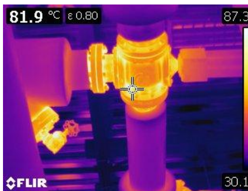
Figure 61 Thermographic image of bare three way valve and strainer at 81° C or 177° F
