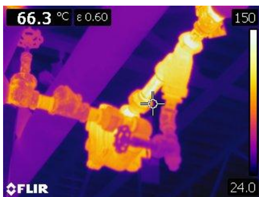
Figure 45 Thermographic image of bare steam trap in the penthouse fan room at 66° C or 150° F.
