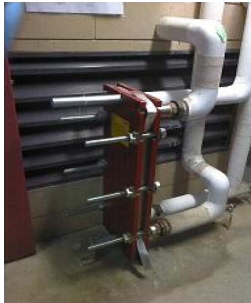
Figure 33 Conventional image of the same plate exchanger.
