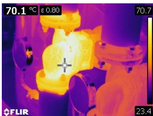
Figure 30 Thermographic image of motorized pumps from hot water tank.
