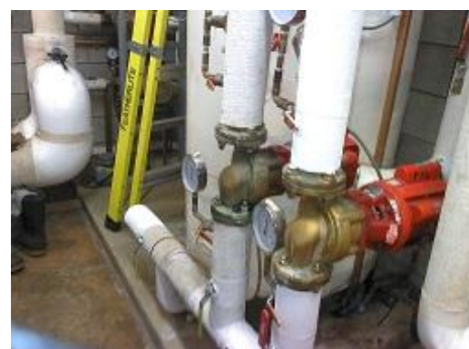
Figure 31 conventional image of the same pumps at the hot water tank.
