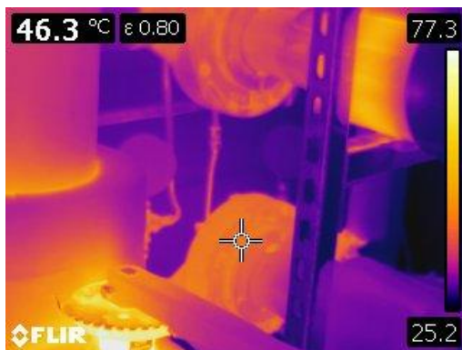
Figure 28 Thermographic image of motorized heating pumps in boiler room.
