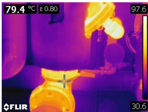
Figure 34 Thermographic image of another motorized heating pump in the boiler room.
