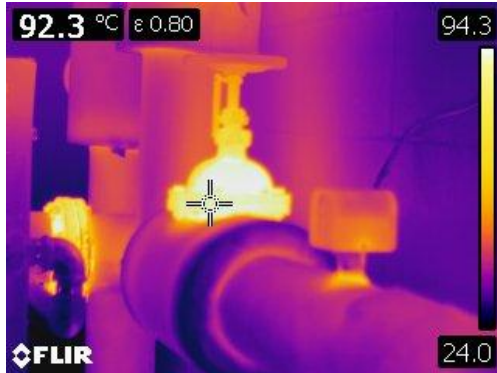
Figure 3 This thermographic image of exposed valve bonnets on the supply line from the E-Plus boiler.
