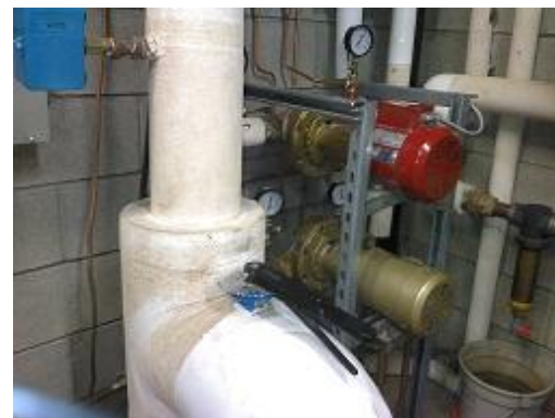
Figure 29 Conventional image of motorized heating pumps in boiler room.
