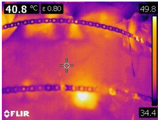
Figure 36 Thermographic image of the domestic hot water tank in boiler room. The insulation is not preventing the necessary heat loss as the surface temperature is 40.8
