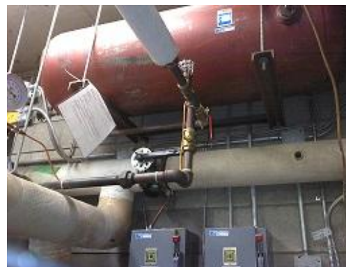
Figure 18 Conventional image of the same 1 inch line with valves and fittings.
