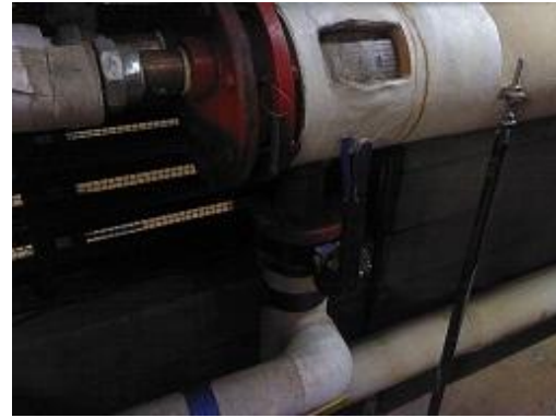
Figure 10 This is the conventional image of the same bare valve in the boiler room.
