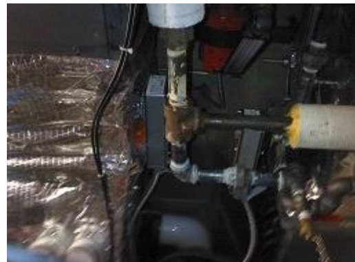
Figure 6 This conventional photo shows the same piping and also shows that the insulation was removed for maintenance.
