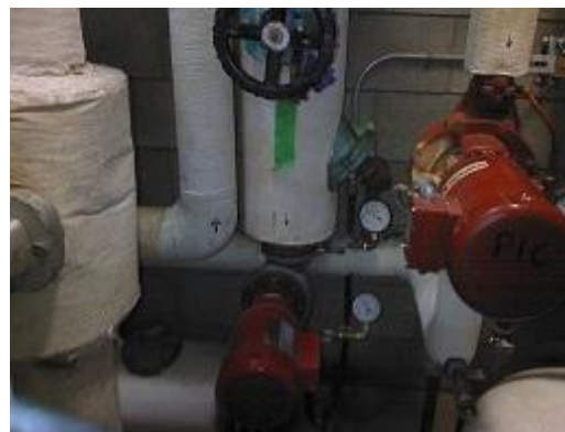
Figure 35 Conventional image of the same motorized pump in the boiler room.
