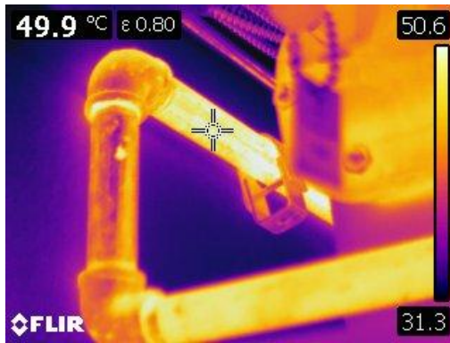
Figure 15 This thermographic image is of a bare 1 inch line adjacent to valve bonnet.
