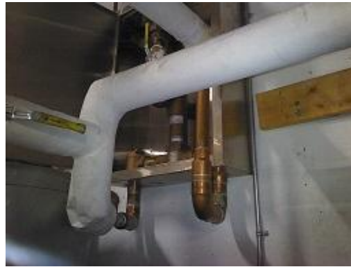
Figure 6 This conventional photo shows the same piping and also shows the deterioration of the mechanical insulation and fittings.
