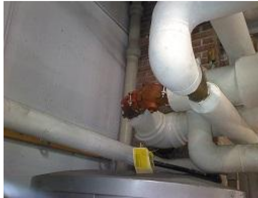
Figure 20 Conventional image of the same elbow and backflow preventer.
