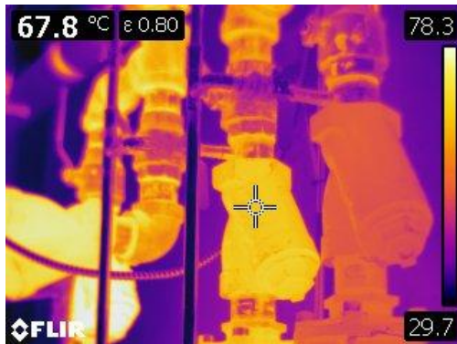
Figure 27 Thermographic image of hanger supports without insulation behind plates.
