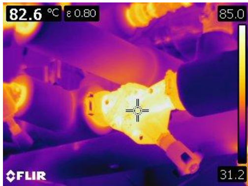
Figure 13 This thermographic image is of a bare control valve.
