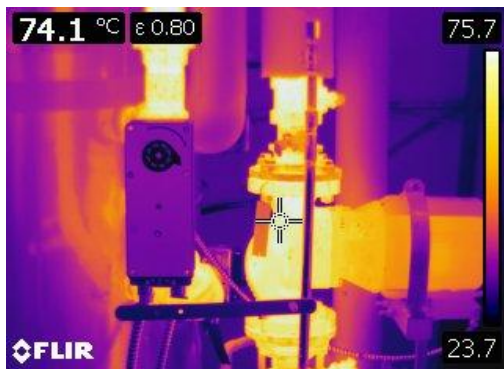
Figure 15 This thermographic image is of a motorized pump from the domestic hot water tank.
