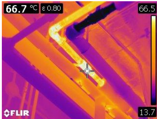
Figure 7 This is a thermographic image of a bare 1 1/4 pipe above the boilers.
