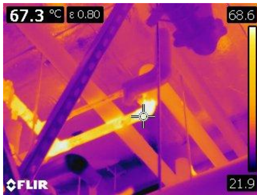
Figure 25 Thermographic image of missing insulation on small bore heating supply.
