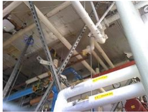
Figure 26 Conventional image of the same piping with damaged and missing insulation.
