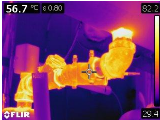
Figure 21 Thermographic image of a control valve, thermostat and elbow from the heating supply line.
