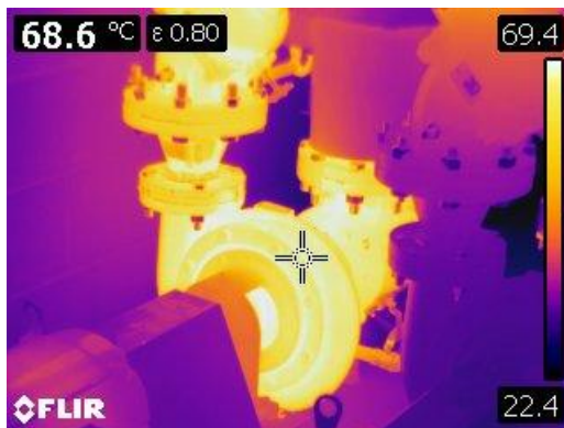
Figure 117 Thermographic image of heating pumps and valves at 68.6° C or 155° F
