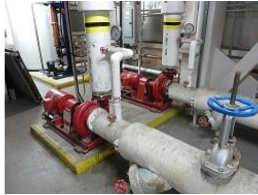
Figure 60 Conventional image of the same heating pumps.
