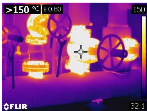
Figure 55 Thermographic image of bare valves on steam header at 150° C or 302° F
