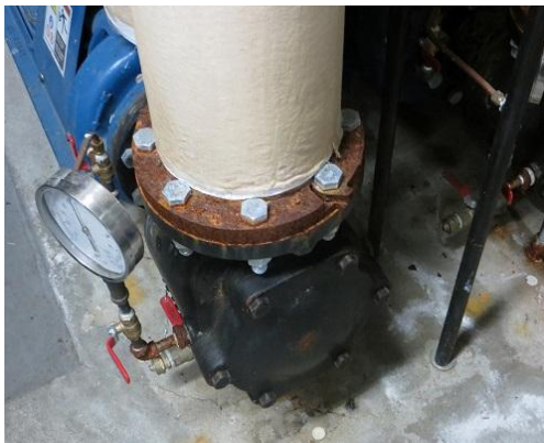
Figure 143 The flange pictured here shows rusting which will allow moisture into the insulation.
