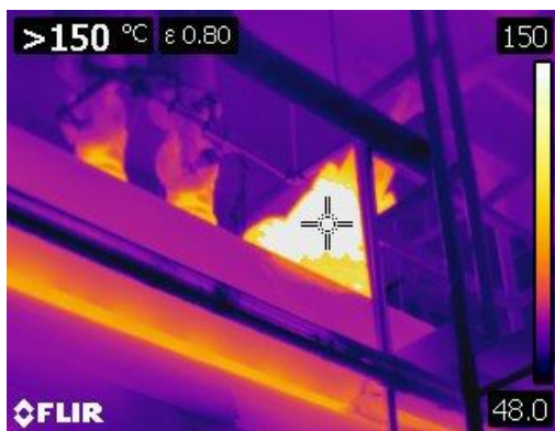
Figure 31 Thermographic image of valves at top of boilers at 150° C or 302° F.
