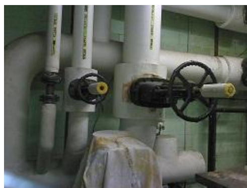
Figure 48 Conventional image of bare vane bonnets.
