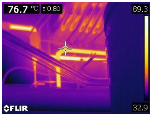
Figure 131 Thermographic image of exposed bare piping at 76.7° C or 170° F
