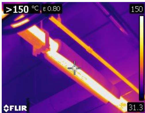
Figure 19 Thermographic image of the bare steam line at 150° C or 302° F
