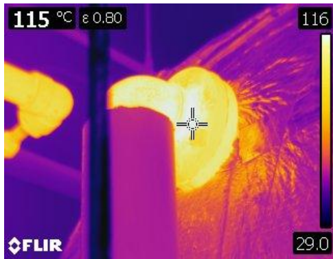
Figure 13 Thermographic image of a bare flange to tank at 115° C or 239° F.
