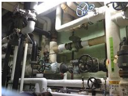
Figure 54 Conventional image of the same pressure reducing valve and other items.
