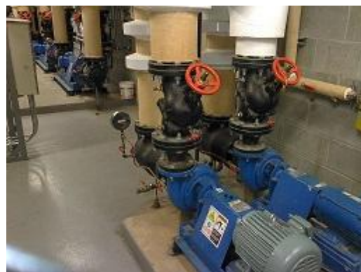
Figure 124 Conventional image of the same heating pumps and valves.
