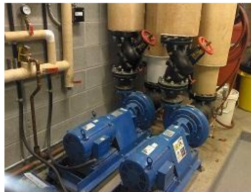
Figure 118 Conventional image of the same heating pumps and valves.
