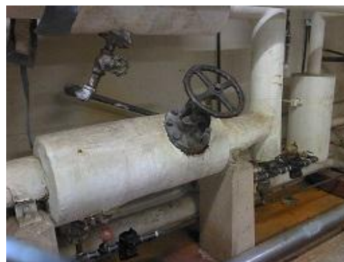
Figure 92 Conventional image of the valve bonnet.
