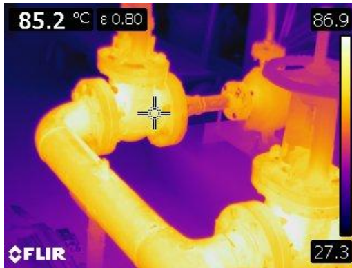
Figure 135 Thermographic image of exposed bare piping and valves at 85.2° C or 185° F
