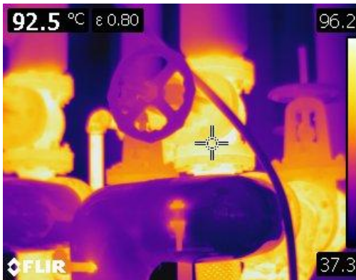
Figure 39 Thermographic image of bare valves and flanges at 92.5° C or 198° F.
