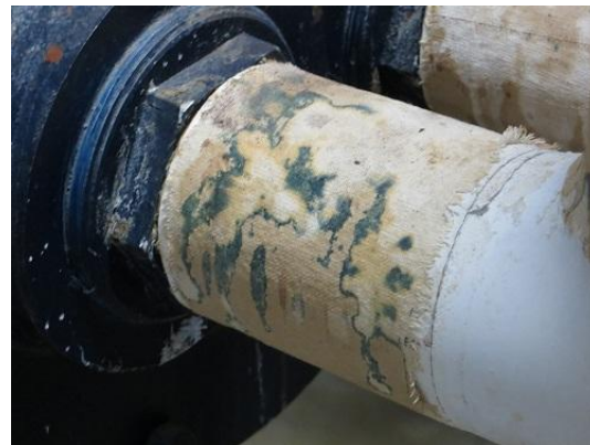
Figure 144 The result of moisture forming on the exposed steel allows for the formation of mold in the canvas. This happening in many areas where vapor barrier is incomplete.
