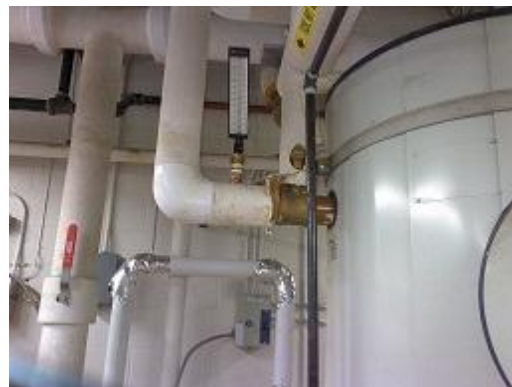
Figure 86 Conventional image of the same missing insulation.
