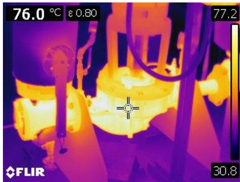
Figure 99 Thermographic image of a motorized heating pump at 76° C or 168° F
