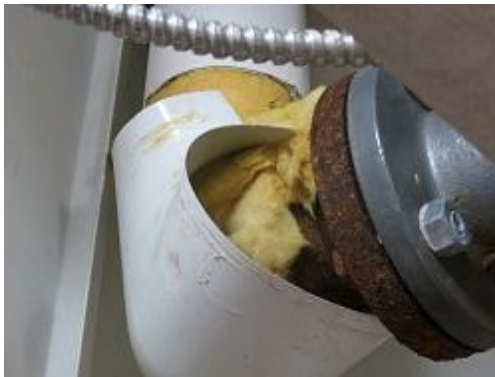
Figure 141 This image shows why an integral vapor barrier is necessary. Lack of a vapor barrier will lead to future corrosion issues.
