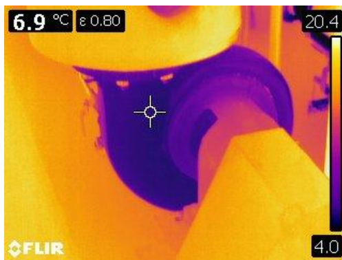
Figure 137 Thermographic image of bare pumps and filter housings which result in condensation and corrosion.
