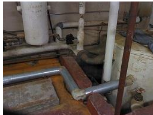
Figure 90 Conventional image of the steam condensate line.
