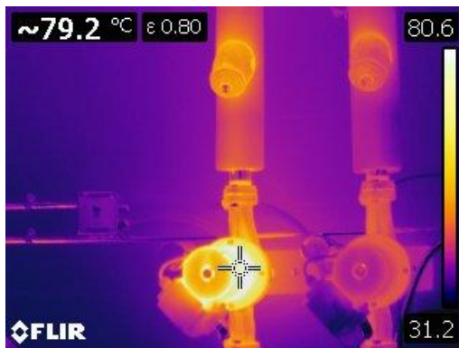
Figure 83 Thermographic image of 2 motorized pumps at hot water tanks at 79.6° C or 175° F
