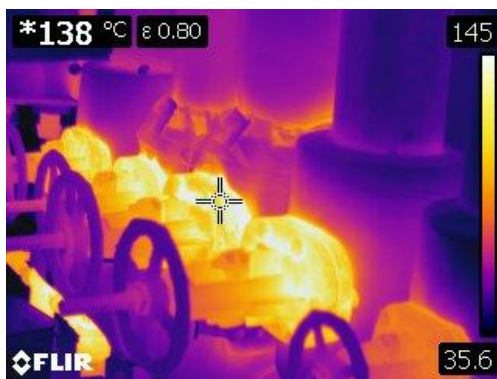
Figure 95 Thermographic image of bare valve bonnets on steam line at 138° C or 280° F
