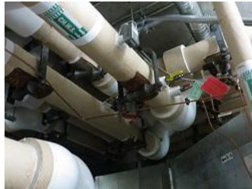
Figure 142 This image shows the wrong use of pipe supports on chilled systems where the vapor barrier is compromised.
