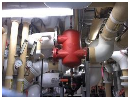
Figure 128 Conventional image of the same expansion tank.
