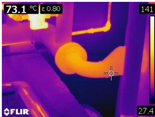
Figure 87 Thermographic image of missing insulation on steam condensate line at 150° C or 302° F
