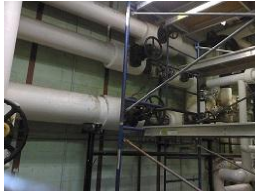
Figure 50 Conventional image of valve bonnets and pressure reducing valve.
