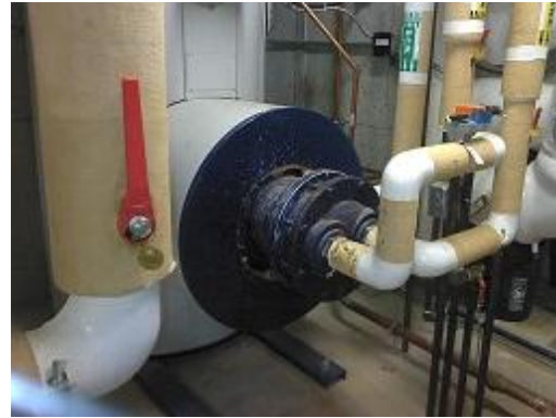
Figure 126 Conventional image of the same heat exchanger and hot water tank.
