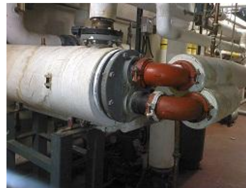
Figure 102 Conventional image of the heat exchanger head and piping.
