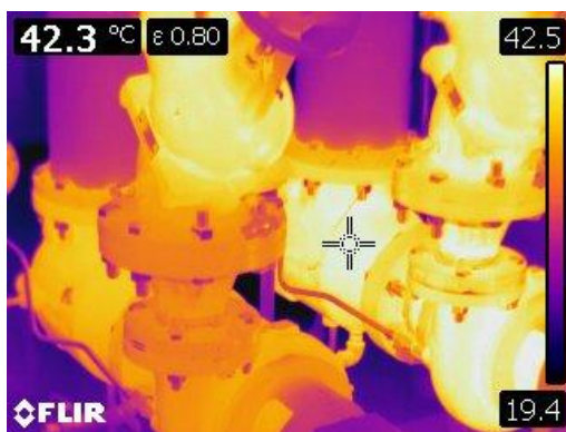
Figure 123 Thermographic image of motorized heating pumps and valves at 42.3° C or 108° F
