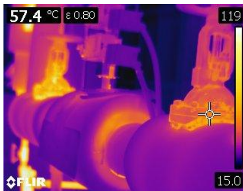
Figure 27 Thermographic image of valve bonnets and piping at 57.4° C or 135° F. -note the heat loss under PVC fitting.
