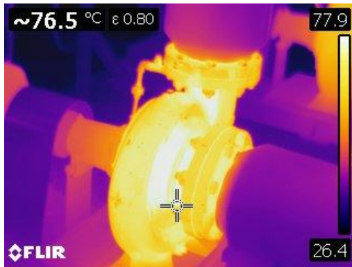
Figure 59 Thermographic image of bare heating supply pump at 76.5° C or 169° F
