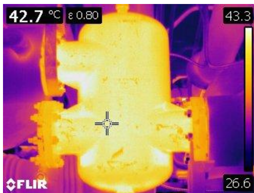
Figure 127 Thermographic image of an expansion tank at 42.7° C or 108° F
