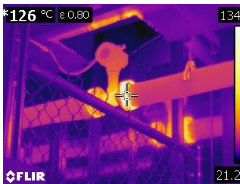
Figure 81 Thermographic image of 2 flow meters at 126° C or 258° F
