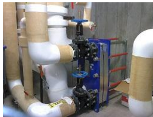
Figure 122 Conventional image of the same heat exchanger and valves.
