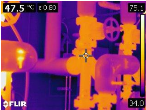
Figure 37 Thermographic image of valves, pumps and piping at 47.5° C or 117° F.
