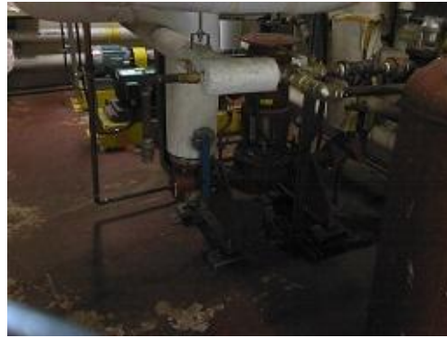
Figure 100 Conventional image of motorized heating pump.
