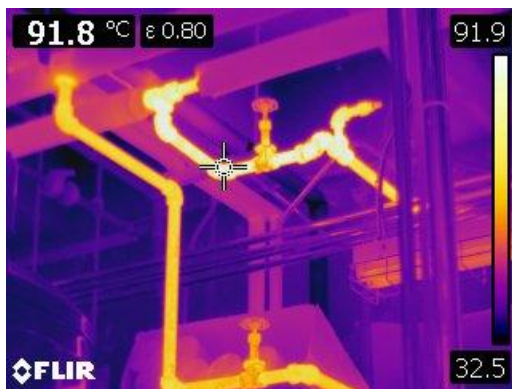
Figure 133 Thermographic image of exposed bare piping at 76.7° C or 170° F
