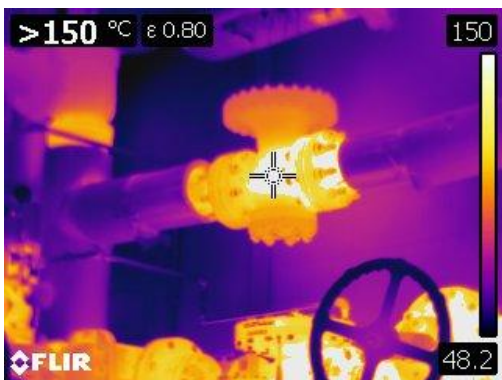
Figure 53 Thermographic image of pressure reducing valve at 150° C or 302° F
