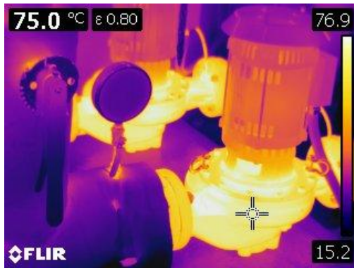
Figure 7 This is a thermographic image of two motorized heating pumps at 75° C or 167° F.
