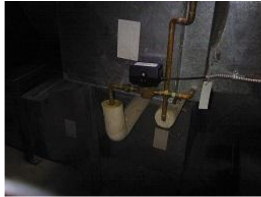
Figure 40 Conventional image of bare small bore heating supply and return to coils.
