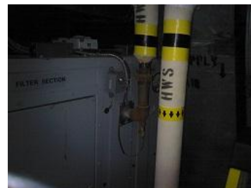
Figure 38 Conventional image of bare small bore heating supply and return to coils.
