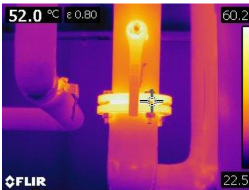
Figure 13 This thermographic image is of bare flange to hot water tanks.
