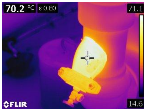
Figure 9 This is a thermographic image of a Victaulic strainer/drain at 70.2° C or 158°F. There is a risk to personnel where temperatures exceed 65 ° C.
