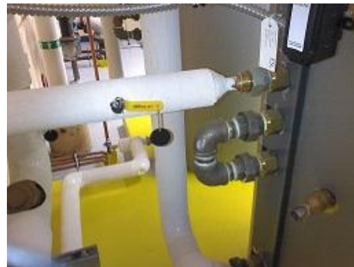
Figure 18 Conventional image of the same by-pass. Note the other bare piping/unions and strainer protruding through the insulation. Each object is a source of heat loss.
