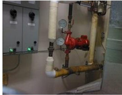
Figure 46 Conventional image of the same small bore supply and return lines and motorized pump.
