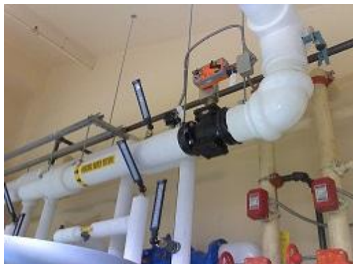
Figure 18 Conventional image of the same by-pass. Note the other bare piping/unions and strainer protruding through the insulation. Each object is a source of heat loss.
