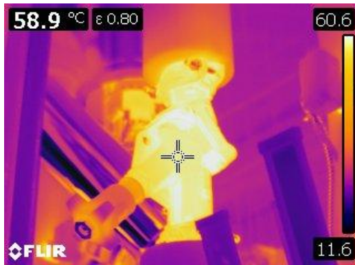
Figure 23 Thermographic image of control valves at the back of the boilers.
