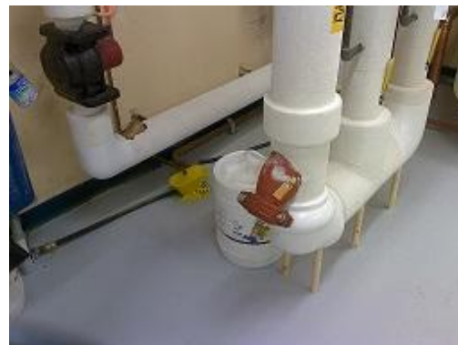
Figure 8 This is a conventional photo of the two heating pumps. These pumps could have removable pads made and installed. The pads are re-useable for maintenance purposes.
