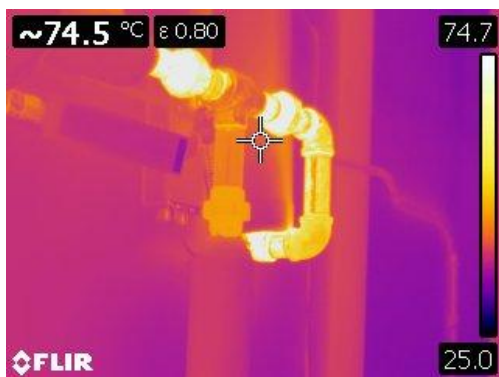
Figure 43 Thermographic image of bare three way small bore supply and return.
