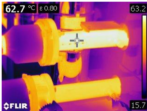
Figure 25 Thermographic image of the supply and return lines at the back of the boiler.
