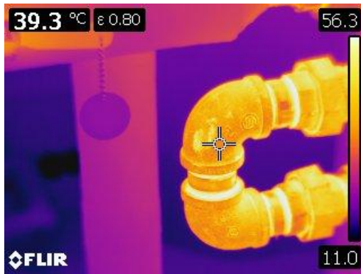
Figure 17 Thermographic image of a by-pass on the back of the boiler.
