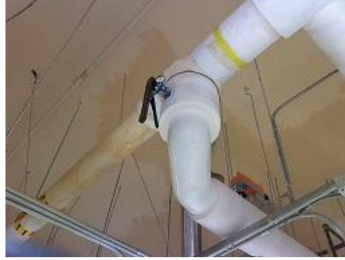
Figure12 This is a conventional image of the same valve and elbow. The thermal image shows the lack of insulation in some areas which is invisible to the naked eye.
