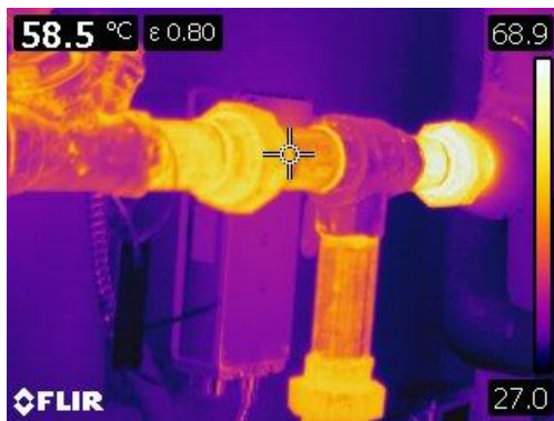
Figure 41 Thermographic image of bare three way small bore supply and return.
