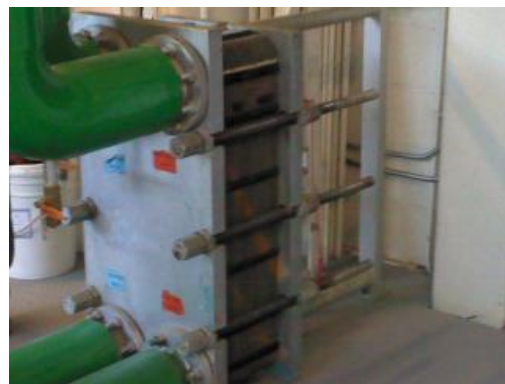
Figure 2 This photo shows the same plate heat exchanger.
