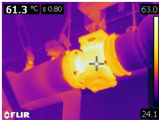
Figure 19 Thermographic image of motorized valve at 61° C or 141° F.
