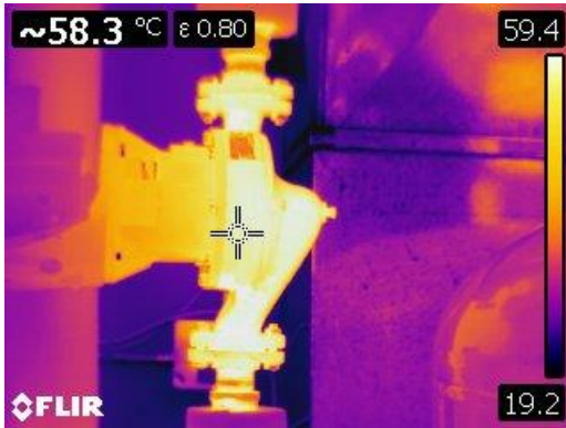
Figure 3 This thermographic image of an exposed motorized heating pump at 58° C or 136° F.
