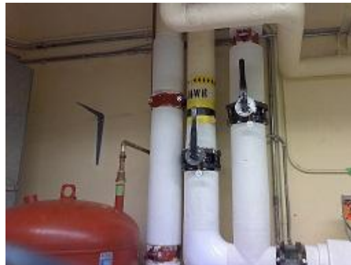
Figure 6 This conventional photo shows the same valves and exposed Victaulic fittings. This work has been recently done and these valves and fittings should have been insulated.
