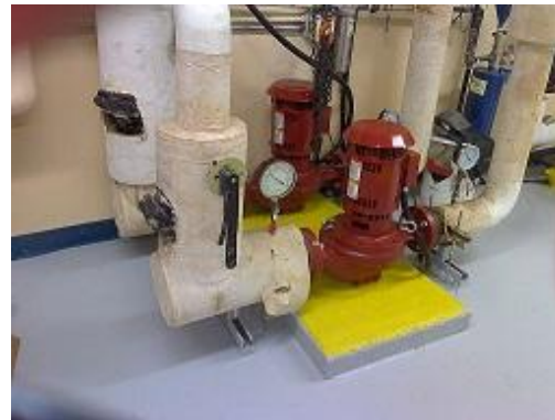
Figure 8 This is a conventional photo of the two heating pumps. These pumps could have removable pads made and installed. The pads are re-useable for maintenance purposes.
