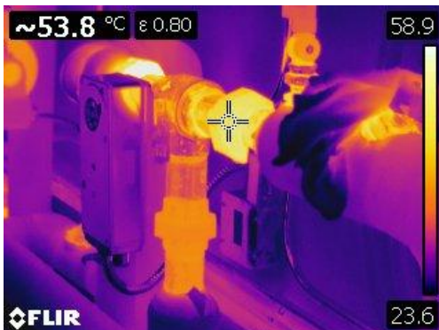
Figure 31 Thermographic image of bare motorized Tee at AHU -1.
