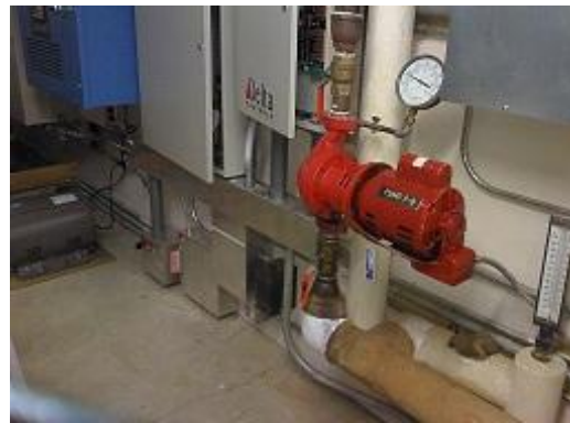
Figure 34 Conventional image of the same motorized heating pump.
