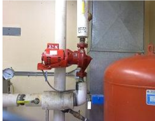
Figure 4 This is a conventional photo of the same pump. There is also an exposed strainer and union.
