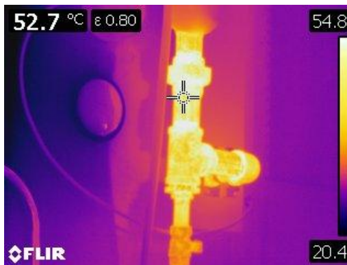
Figure 33 Thermographic image of bare motorized heating pump P-1.
