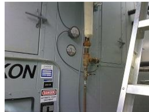
Figure 36 Conventional image of bare small bore heating supply to coils.
