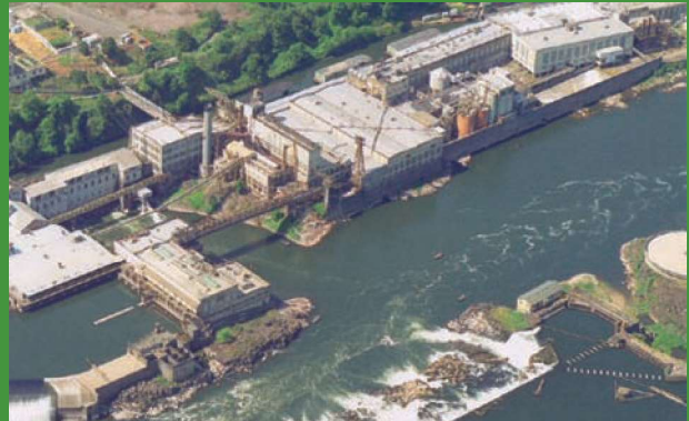
Steam is used to dry paper and power two papermaking machines at the West Linn Paper Company's mill in West Linn, Oregon, which produces nearly 700 tons daily of coated paper.
