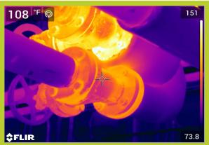
Operating Temperature, Ambient Temperature, Insulation selected 150\*F 65\*F Fiberglass Emittance of Surface
