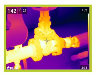
Operating Temperature, Ambient Temperature, Insulation selected 154\*F 65\*F Fiberglass Emittance of Surface
