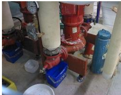
Figure 32 Conventional image of the same heating pumps.
