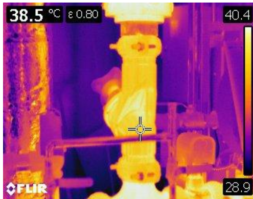
Figure 75 Thermographic image of control valve and piping at boiler.
