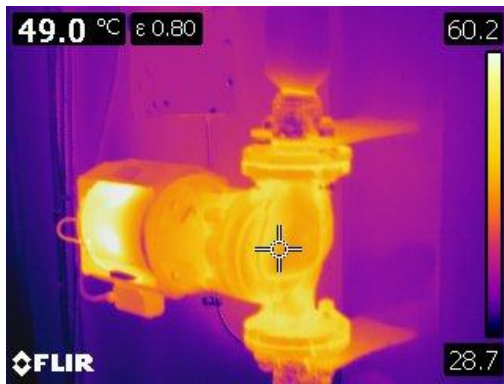
Figure 81 Thermo graphic image of heating pump and associated piping.
