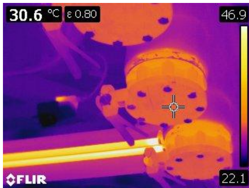
Figure 35 Thermographic image of the exposed gate valves on the Thermonex header.
