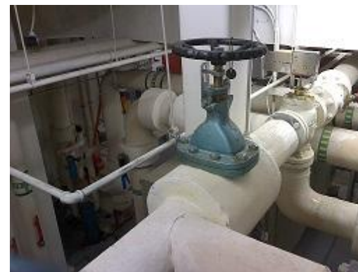
Figure 62 Conventional image of exposed valve bonnet and other exposed valves and flanges.
