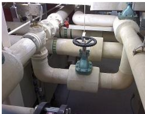
Figure 64 Conventional image of exposed valve bonnet and other exposed valves and flanges.
