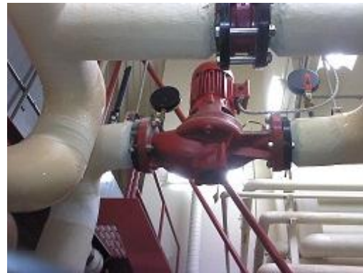
Figure 60 Conventional picture of exposed heating pump.
