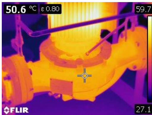
Figure 77 Thermographic image of heating pump and associated piping.
