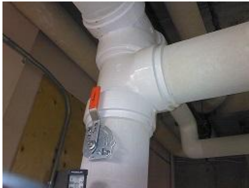
Figure 6 This conventional photo shows the PVC fitting applied to the Victaulic Tee. The fitting looks great but the thermographic image shows a high rate of heat loss.
