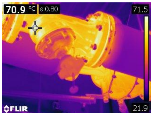
Figure 25 Thermographic image of three way valve requiring insulation.
