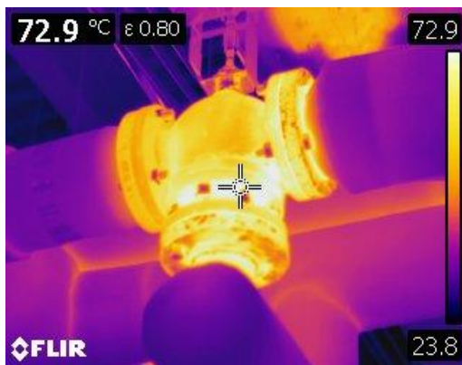
Figure 25 Thermographic image of three way valve requiring insulation.
