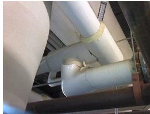
Figure 48 Conventional image of the same pipe covering and elbow with heat loss at intersection of materials.
