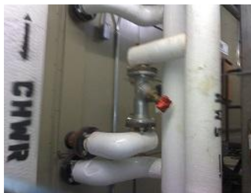
Figure 58 Conventional picture of exposed control valve and flanges to unit.
