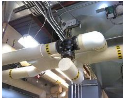
Figure 26 Conventional image of the same valve and flanges requiring insulation.
