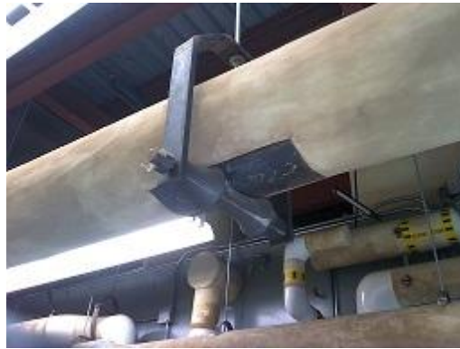
Figure 30 Conventional picture of hanger support.
