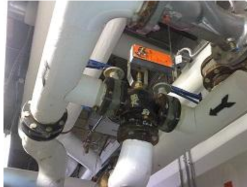
Figure 58 Conventional image of exposed three way valve.
