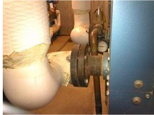
Figure 54 Conventional image of exposed flanges.
