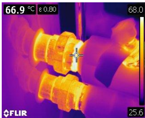
Figure 9 This is a thermographic image of the supply and return lines at the back of the boiler. These two lines are operating at a high temperature and pose a personal protection hazard.
