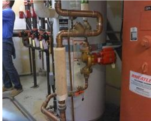
Figure 20 Conventional image of the pump adjacent to the domestic hot water tank.
