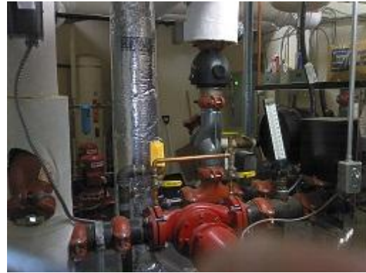
Figure 76 Conventional picture of bare valves, pumps and piping.
