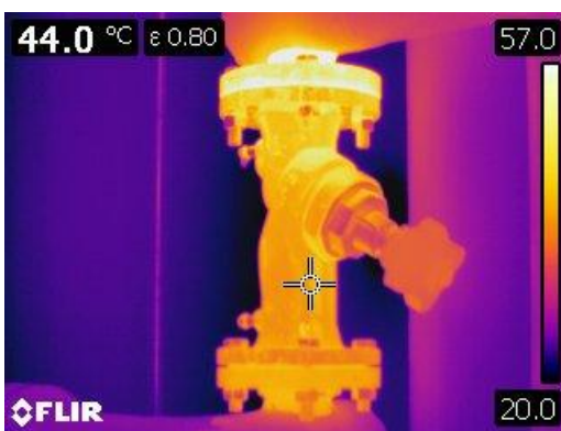
Figure 57 Thermographic image of exposed control valve.
