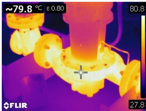
Figure 43 Thermographic image of exposed heating pump.
