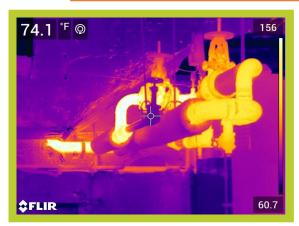
Operating Temperature, Ambient Temperature, Insulation selected 156\*F 75\*F Fiberglass Emittance of Surface
