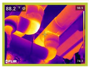
Operating Temperature, Ambient Temperature, Insulation selected 97\*F 75\*F Fiberglass Emittance of Surface
