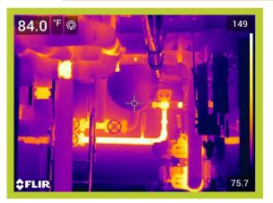
Operating Temperature, Ambient Temperature, Insulation selected 149\*F 75\*F Fiberglass Emittance of Surface
