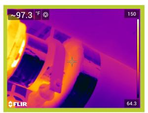
Operating Temperature, Ambient Temperature, Insulation selected 94\*F 74\*F Fiberglass Emittance of Surface
