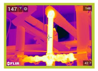
Operating Temperature, Ambient Temperature, Insulation selected 140\*F 75\*F Fiberglass Emittance of Surface Expected Useful Life of Insulation System Operating hours per year Efficiency of fuel Conversion%
