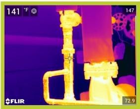
Operating Temperature, Ambient Temperature, Insulation selected 140\*F 76 F Fiberglass Emittance of Surface Expected Useful Life of Insulation System Operating hours per year Efficiency of fuel Conversion%
