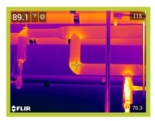
Operating Temperature, Ambient Temperature, Insulation selected 110\*F 74\*F Fiberglass Emittance of Surface
