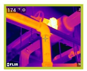
Operating Temperature, Ambient Temperature, Insulation selected 175\*F 81\*F Fiberglass Emittance of Surface0.95Expected Useful Life of Insulation System20 yrs.Operating hours per year8320Efficiency of fuel Conversion%75%
