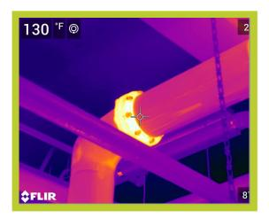
Operating Temperature, Ambient Temperature, Insulation selected 235\*F 81\*F Fiberglass Emittance of Surface
