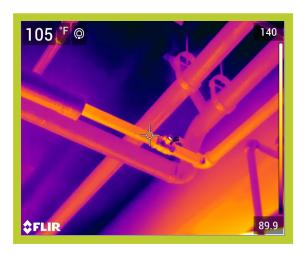
Operating Temperature, Ambient Temperature, Insulation selected 104\*F 81\*F Fiberglass Emittance of Surface0.95Expected Useful Life of Insulation System20 yrs.Operating hours per year8320Efficiency of fuel Conversion%75%
