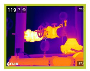
Operating Temperature, Ambient Temperature, Insulation selected 176\*F 81\*F Fiberglass
