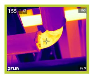
Operating Temperature, Ambient Temperature, Insulation selected 156\*F 81\*F Fiberglass Emittance of Surface Expected Useful Life of Insulation System Operating hours per year Efficiency of fuel Conversion%
