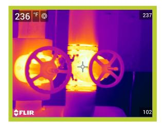
Operating Temperature, Ambient Temperature, Insulation selected 230\*F 88\*F Fiberglass
