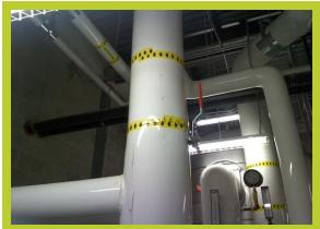
Operating Temperature, \*F Ambient Temperature, \*F Insulation selected 194 78 Fiberglass Emittance of Surface 0.95
