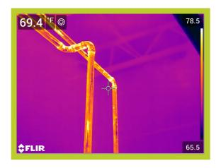
Operating Temperature, Ambient Temperature, Insulation selected 120\*F 69\*F Fiberglass Emittance of Surface Expected Useful Life of Insulation System Operating hours per year Efficiency of fuel Conversion%
