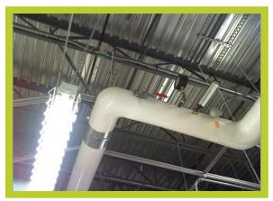
Operating Temperature, \*F Ambient Temperature, \*F Insulation selected 158 80 Fiberglass Emittance of Surface 0.95
