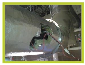
Operating Temperature, \*F Ambient Temperature, \*F Insulation selected 302 78 Mineral Wool Emittance of Surface
