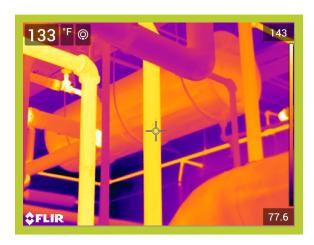
Operating Temperature, Ambient Temperature, Insulation selected 142\*F 70\*F Fiberglass Emittance of Surface Expected Useful Life of Insulation System Operating hours per year Efficiency of fuel Conversion%
