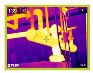
Operating Temperature, Ambient Temperature, Insulation selected 136\*F 70\*F Fiberglass
