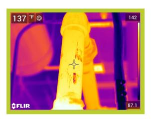
Operating Temperature, Ambient Temperature, Insulation selected 141\*F 70\*F Fiberglass
