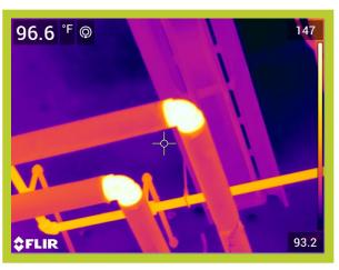
Operating Temperature, Ambient Temperature, Insulation selected 123\*F 70\*F Fiberglass Emittance of Surface
