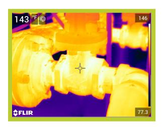
Operating Temperature, Ambient Temperature, Insulation selected 145\*F 70\*F Fiberglass
