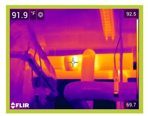
Operating Temperature, Ambient Temperature, Insulation selected 92 \*F 68 \*F Fiberglass
