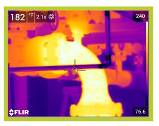
Operating Temperature, Ambient Temperature, Insulation selected 240\*F 81\*F Fiberglass
