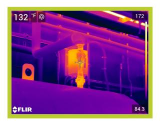
Operating Temperature, Ambient Temperature, Insulation selected 130\*F 81 \*F Fiberglass Emittance of Surface0.95Expected Useful Life of Insulation System20 yrs.Operating hours per year8320Efficiency of fuel Conversion%75%
