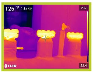
Operating Temperature, Ambient Temperature, Insulation selected 232\*F 81\*F Fiberglass Emittance of Surface
