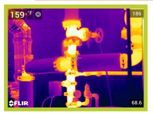
Operating Temperature, Ambient Temperature, Insulation selected 168\*F 67\*F Fiberglass Emittance of Surface Expected Useful Life of Insulation System Operating hours per year Efficiency of fuel Conversion% 0.95 20 yrs. 8760 85%
