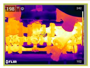
Operating Temperature, Ambient Temperature, Insulation selected 225\*F 73\*F Fiberglass Emittance of Surface
