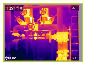
Operating Temperature, Ambient Temperature, Insulation selected 185\*F 71\*F Fiberglass
