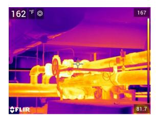
Operating Temperature, Ambient Temperature, Insulation selected 165\*F 77\*F Fiberglass
