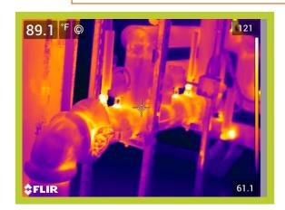
Operating Temperature, Ambient Temperature, Insulation selected 155\*F 62\*F Fiberglass Emittance of Surface0.95Expected Useful Life of Insulation System20 yrs.Operating hours per year8760Efficiency of fuel Conversion%85%
