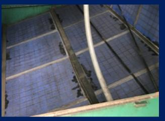
Clogged filters with signs of mold growth
