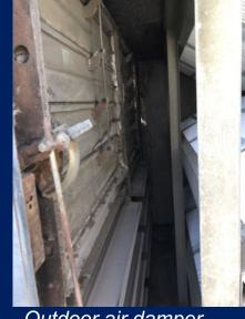
Outdoor air damper shut with actuator removed
