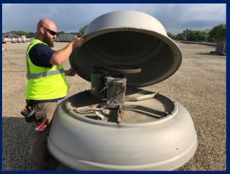
Broken belt on exhaust fan
