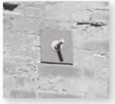
A steel plate with anchor bolts.
