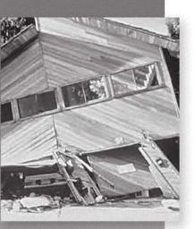
The walls around the garage door of this home were not strong enough to withstand the shaking of the 1989 Loma Prieta Earthquake.
