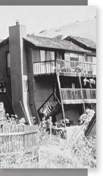
The balcony of this hillside home partially collapsed and the home tilted when the stilt-type support posts and poorly braced walls shifted during an earthquake.
