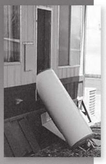
During an earthquake, an unbraced water heater can topple, which can start a fire or lead to major water damage.
