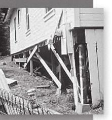
This home's pier-and-post foundation was damaged during an earthquake. The diagonal bracing was added after the earthquake to temporarily stabilize the home during repairs.
