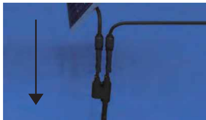
Connection with IP67 coupler
