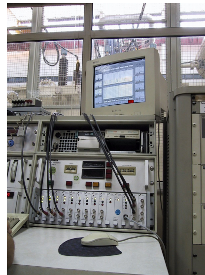
Multi-channel ICMsystem installed in a control room
