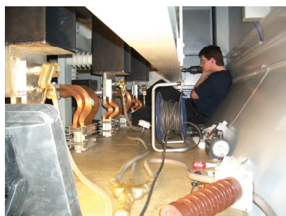
Installing couplers on site
