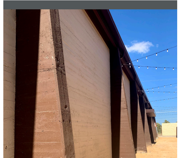
Nineteen buttresses with unique imprints on the concrete needed repair at Wursthalle
