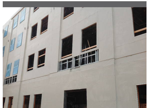
Air barrier installed on one of the residential buildings.
