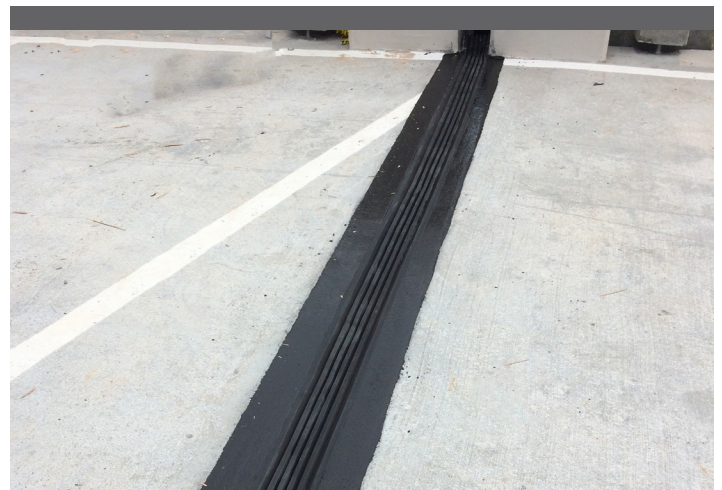
Expansion joint installed in the parking garage.
