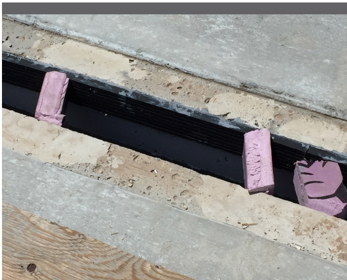
A 3/4-inch gap reducer installed on the wall of the joint with an epoxy adhesive.
