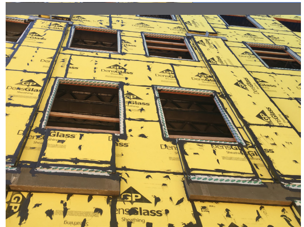
Chamberlin crews sealed the sheathing seams and covered the countersunk screw heads to prevent water from penetrating the building.
