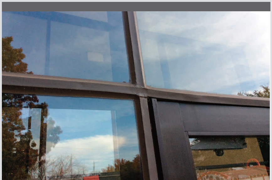
Figure 2: Repaired lock-strip gasket. Photo courtesy of Chamberlin Roofing & Waterproofing.
