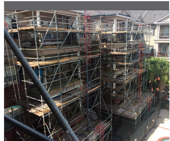
Scaffolding system used to repair and replace damaged balconies at The Buckingham.
