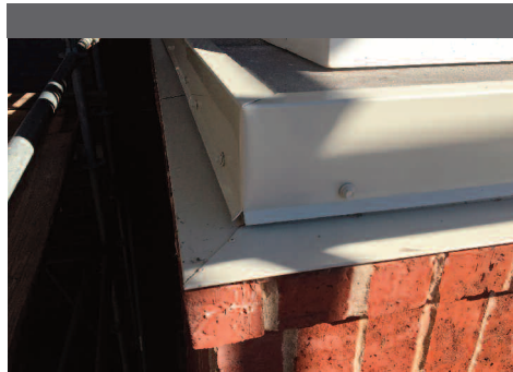
Perimeter retainer metal protecting the waterproofing and pavers.
