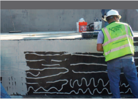
Figure 5: Retroactive sealant application to repair pinholes.
