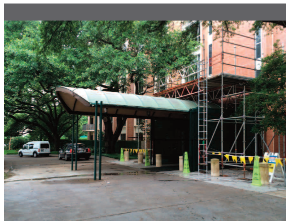
The front entrance of The Hallmark with overhead protection and safety barricades in place.
