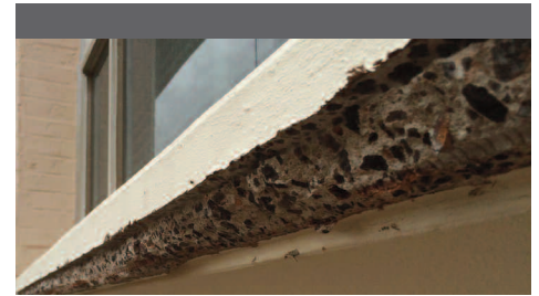
Horizontal eyebrow on the building prepped for concrete patchwork to repair extensive deterioration.
