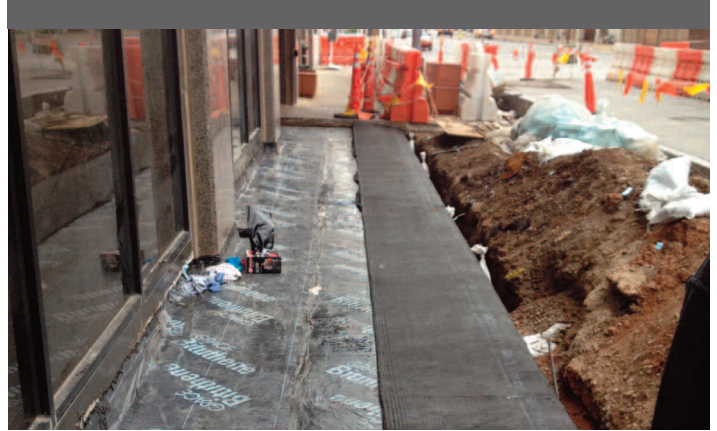
Chamberlin applied waterproofing on multiple sidewalks for Project 180.
