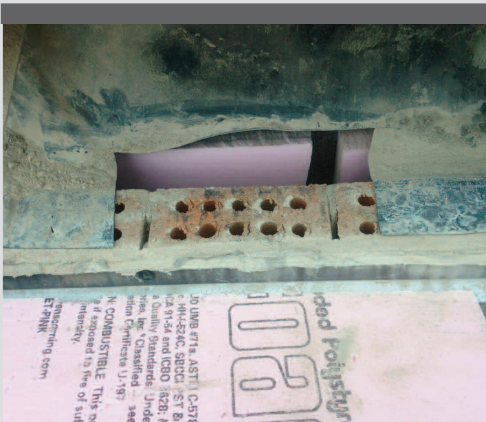
Excavation at a cut back flashing prior to remediation. The flashing installation was a significant source of water infiltration since original construction.
