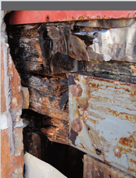
Deterioration of a glulam beam due to improper integration of balcony and wall interface detailing.
