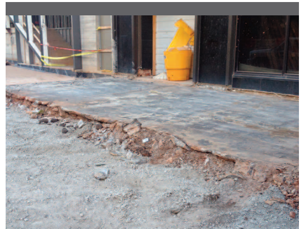
The concrete on the sidewalk and above the basement was severely damaged.
