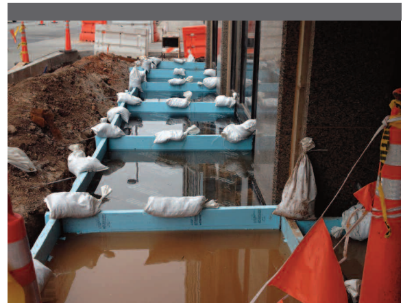
Chamberlin performed water tests to ensure there were no leaks to the underground basement.
