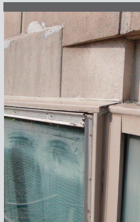
Sloped EIFS and window assemblies, vertical and horizontal offsets. The epitome of complexity, poor detailing, and pushing performance limits. Surprise. It leaked and wasn't durable.
