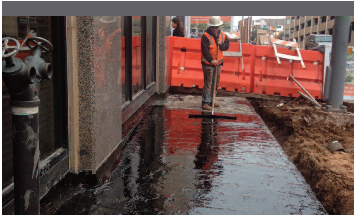
Chamberlin crew member applies a cementitious filler to ensure the waterproofing would be installed properly and adhere to the substrate.
