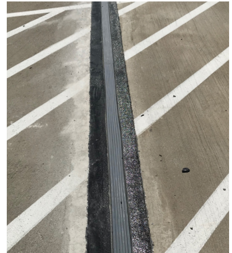
Completed Silspec RFS expansion joint
