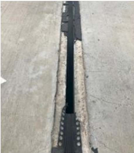
Original wing joint before restoration
