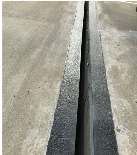
Epoxy nosing to fill in blockouts
