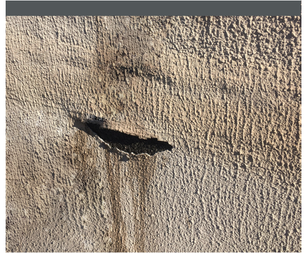
Before and after: Chamberlin cleaned the building envelope and restored the weathered, delaminated existing coating with a new elastomeric coating.
