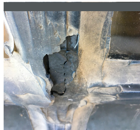
The window gasket system was severely deteriorated in some areas, allowing possible locations for water intrusion.
