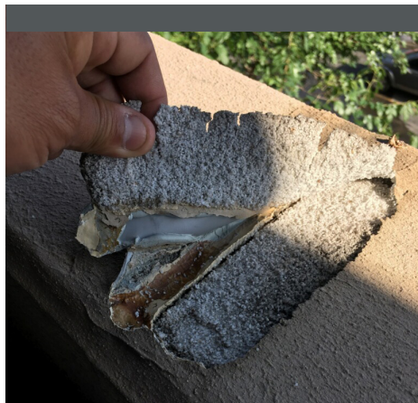
Chamberlin repaired failing joint tape in the parking garage and applied an elastomeric coating.
