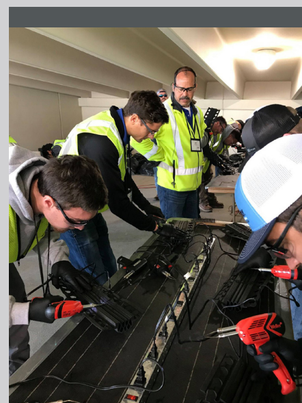
Field slicing of a winged expansion joint seal training.
