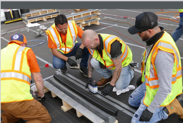
Preparing for a field inflatable expansion joint seal installation.
