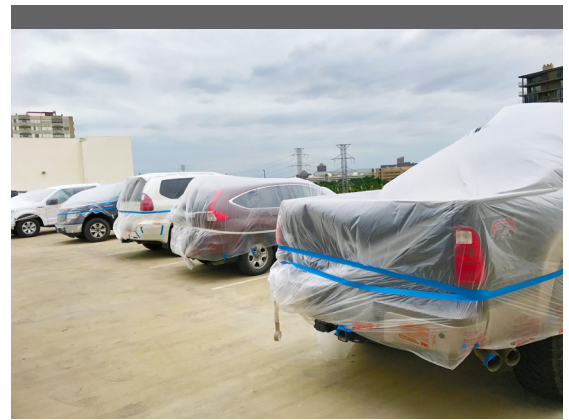
Tarps covered windows, railings, cars and other objects in the surrounding area to protect them from contact with the silicone coating used for the building envelope restoration.
