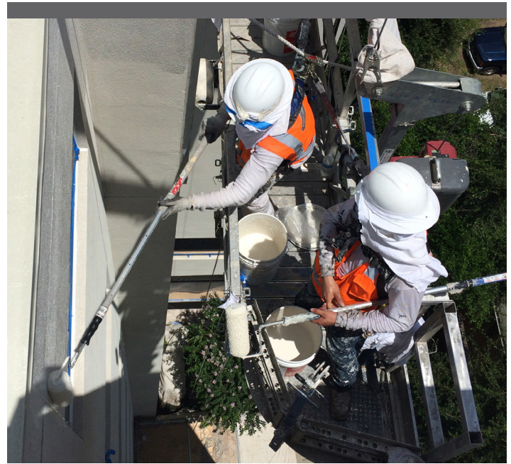
Installation of GE SilShield 2400 for the building envelope restoration on Gables Uptown Trail in Dallas, Texas.
