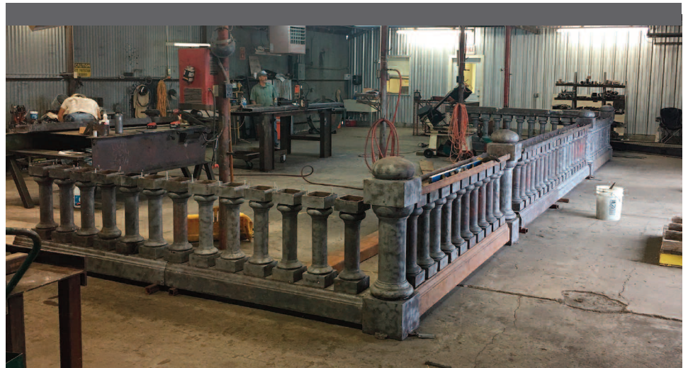
The balustrades were sandblasted to remove the paint and expose cracks before welding.
