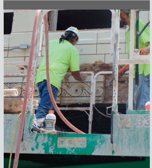
Figure 5: Frequent visits to the site allowed for opportunities to observe and provide alternate strategy for removal of the terra cotta.
