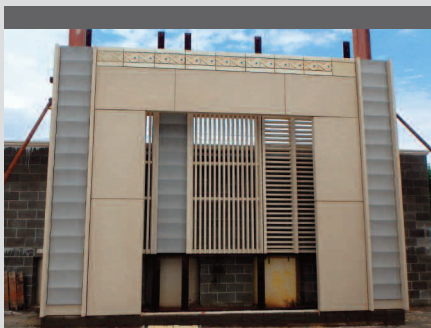
Figure 6: Full scale mock-up of the terra cotta frieze installed into the GFRC panel (note that the end pieces were recreated units being reviewed for acceptance in the final installation).
