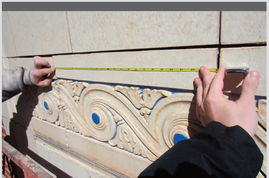
Figure 2: Measurements of the polychromatic terra cotta units and total quantities were made to determine the available quantity for the reinstallation.
