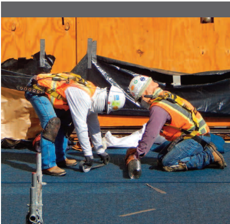
The Chamberlin crew preparing for Electronic Leak Detection (ELD) testing on the waterproofing membrane.
