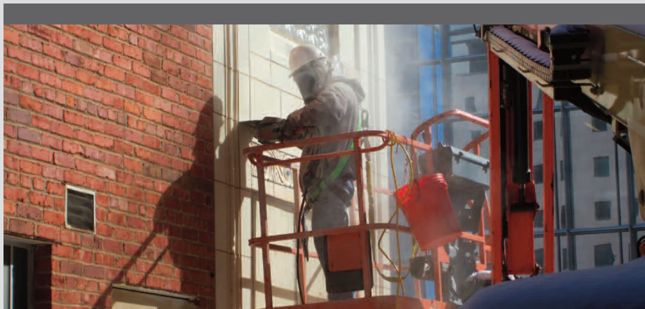
Figure 3: Selective removal and exploratory openings during the investigation were used to determine the type of connection of the terra cotta to the back-up wall.
