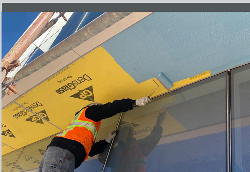
Installation of fluid-applied air barrier with hand roller at computer software office building in Austin, Texas. Photo courtesy of Chamberlin Roofing & Waterproofing.
