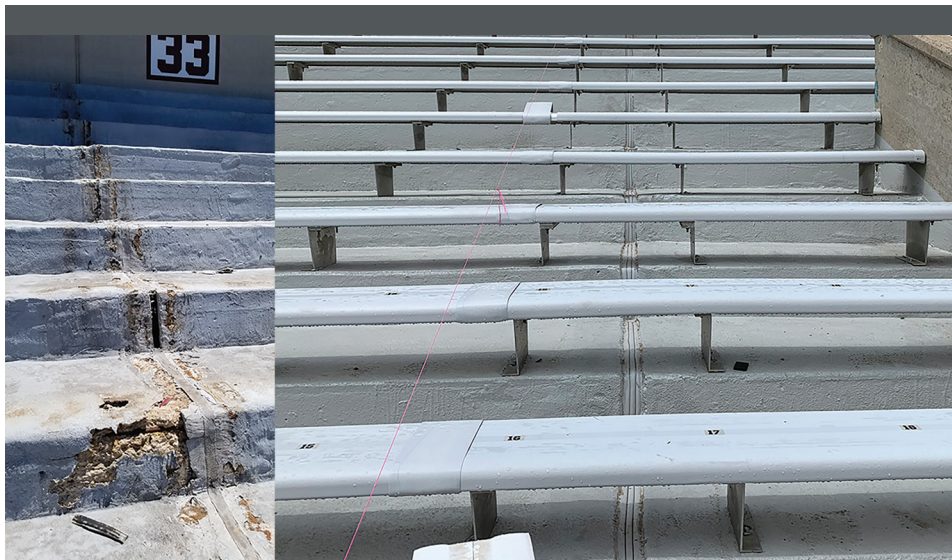
Before and after: Chamberlin remedied expansion joints in the OU stadium to stop water intrusion.
