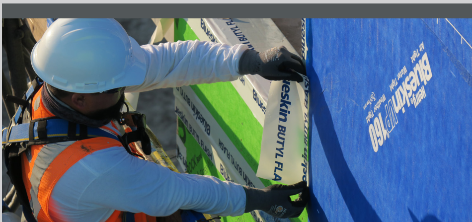
Installation of flashing on a self-adhered vapor permeable, water resistive air barrier membrane in Dallas, Texas. Photo courtesy of Chamberlin Roofing & Waterproofing.
