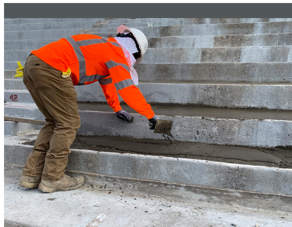
Chamberlin crew member patching concrete prior to traffic coating installation.
