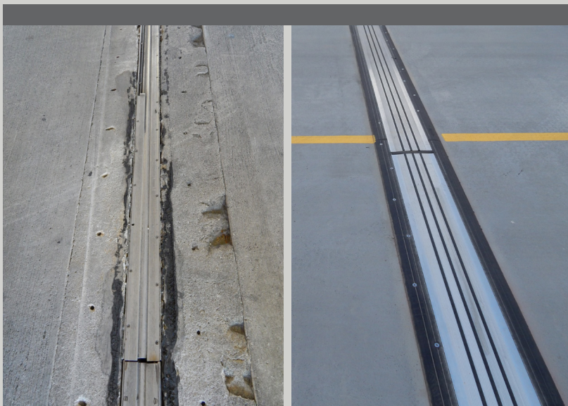
Before and after parking garage expansion joint replacement and traffic coating installation. Photo provided by Chamberlin Roofing & Waterproofing.
