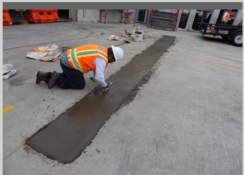
Parking garage concrete repair. Photo provided by Chamberlin Roofing & Waterproofing.
