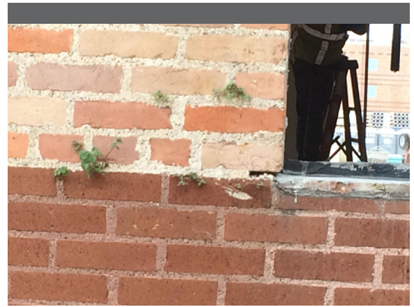
Aged and weathered masonry and mortar in need of repairs and replacements.
