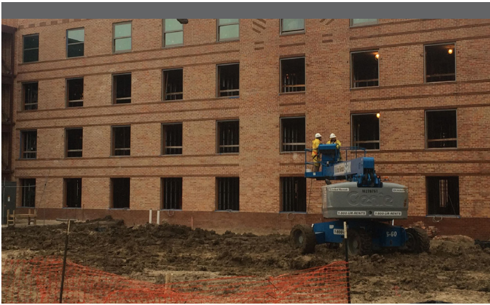
Chamberlin crews secured bricks matching original construction and took care to keep with existing installation patterns during repair and replacement.
