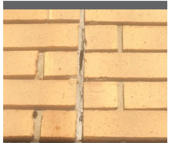
Aged and weathered masonry and mortar in need of repairs and replacements.
