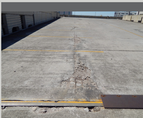
Before and after parking garage concrete patching and traffic coating installation. Photo provided by Chamberlin Roofing & Waterproofing.
