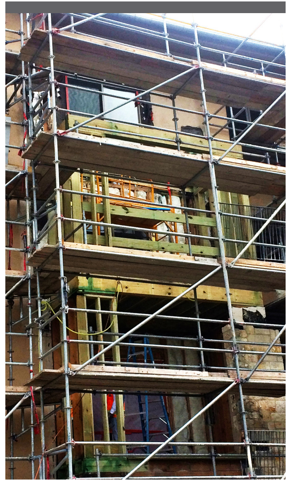
Four stacks of balconies had to be completely demolished and rebuilt.
