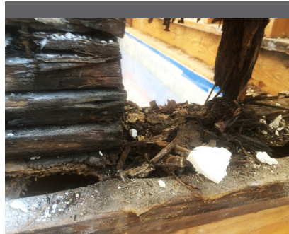
Unforeseen extensive wood rot was found on the balcony decks.
