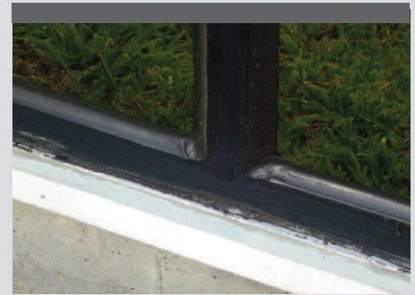
Figure 5: Lock-strip wet sealed
