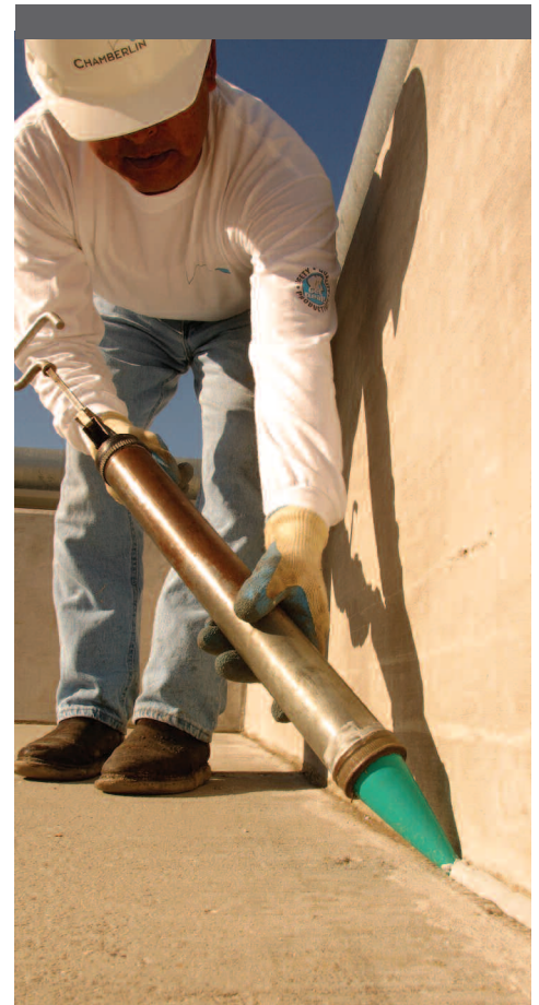
Installation of parking garage joint sealants.
