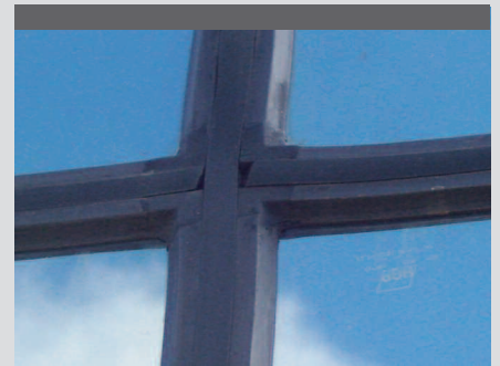
Figure 6: Lock-strip gasket corner
