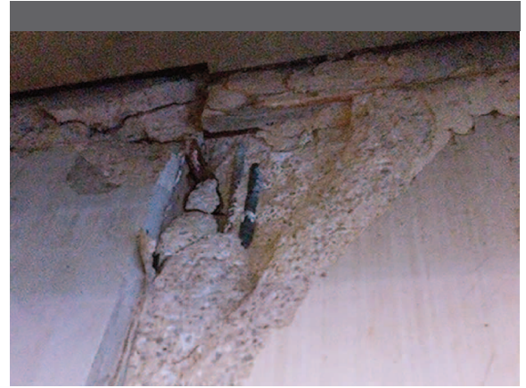
The concrete in the parking garage had sustained extensive corrosion and damage.
