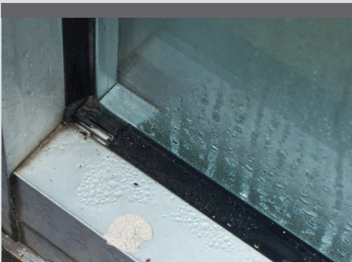
Figure 1: Short gasket at corner of frame
