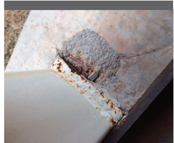
While performing embed repairs, rust was discovered on the rebar.
