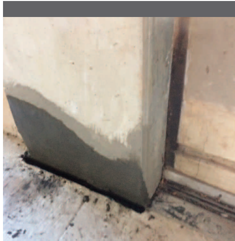
This picture shows an area of concrete patched on a column during the curing process.
