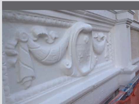
Figure 5: New cast stone spandrel panel installed.
