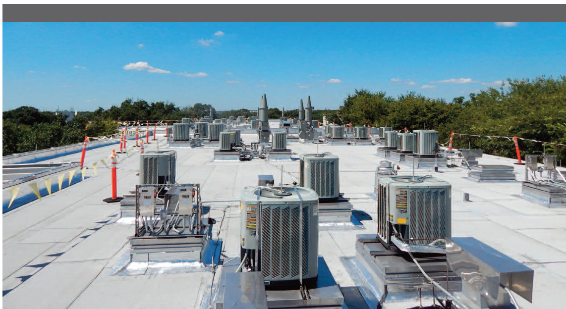
The completed torch-applied roofing system for a leading environmental agency's headquarters in Austin, TX.
