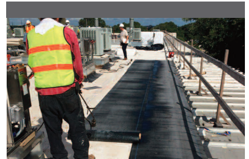
A guardrail system was built on the north side of the roof where there was no parapet wall.
