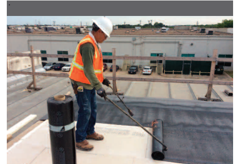
Chamberlin installed 25,000 square feet of torch-applied roofing system.
