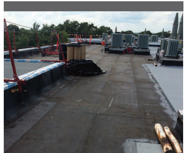
Parapet clamps were used as one fall protection method while the base sheet and cap sheet were being installed.
