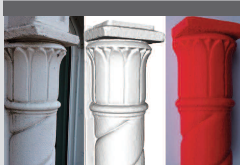
Figure 4: Left - Existing decorative column, Middle - 3D model of column, Right - 3D print of model.
