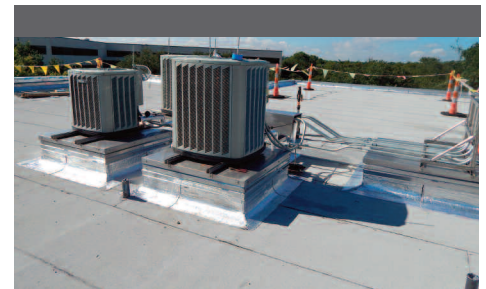
The HVAC units were flashed to keep the building watertight.
