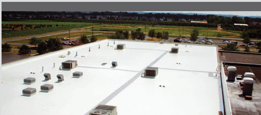
The use of white thermoplastic materials result in lower roof surface temperatures during the summer months when compared to dark colored roofs.
