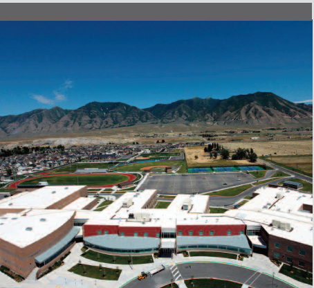
LBNL estimates that the use of cool roofing materials on 80 percent of U.S. commercial buildings would result in 10,400 GWh of cooling energy savings and approximately $735 million in overall energy savings.
