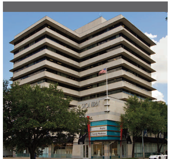
The Art Deco style of the Kirby buildings feature “eyebrow” architectural elements on the entire facade which created unique renovation challenges.
