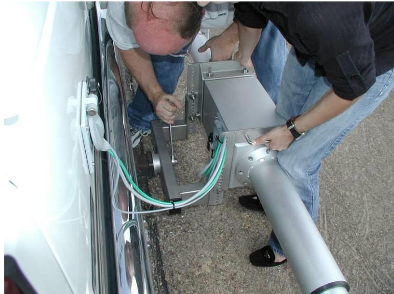
*Figure 27 - Tightening the Mounting Bolt*
