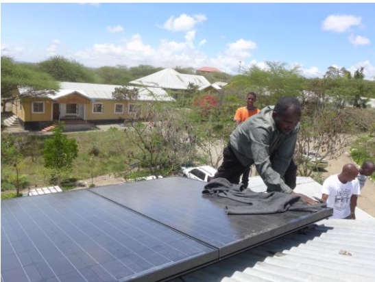
The Climate Fund: Installing solar panels on a school in Northern Tanzania
