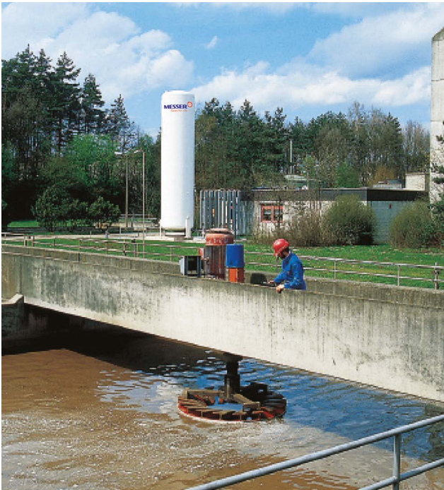
Pure oxygen supports aeration of activated sludge tank
