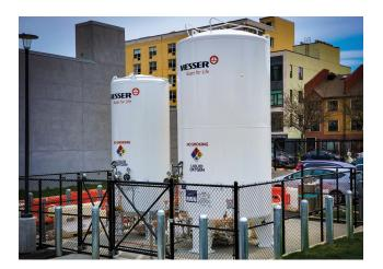
vaporizer(s) appropriate for the healthcare facility's oxygen usage patterns, a local alarm panel for monitoring, and a manifold to regulate  $O_2$  to the hospital.
