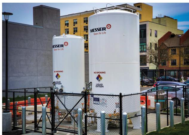
vaporizer(s) appropriate for the healthcare facility's oxygen usage patterns, a local alarm panel for monitoring, and a manifold to regulate O<sub>2</sub> to the hospital.
