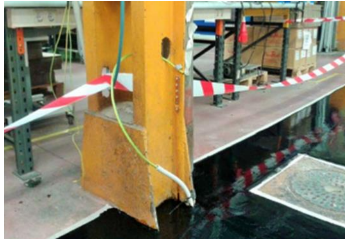
Connecting the ground to the superconducting layer MasterTop P 687 W AS
