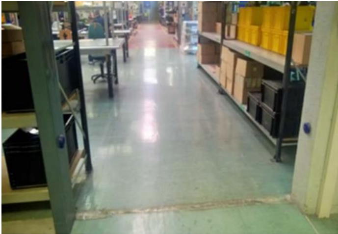
Appearance of the workshop prior to the pavement renovation
