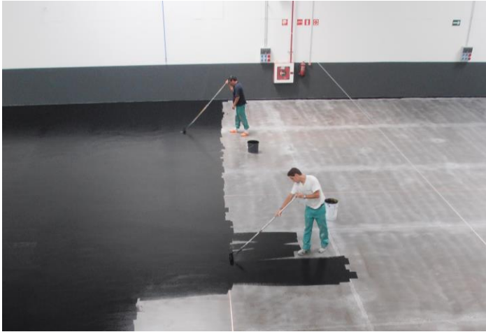
Application of superconductive layer MasterTop P 687 W AS
