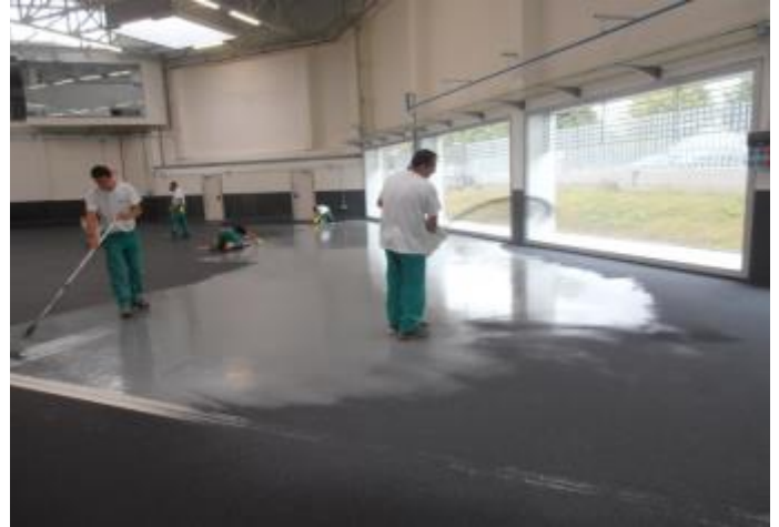
MasterTop BC 370 AS and broadcasting of onductive aggregate
